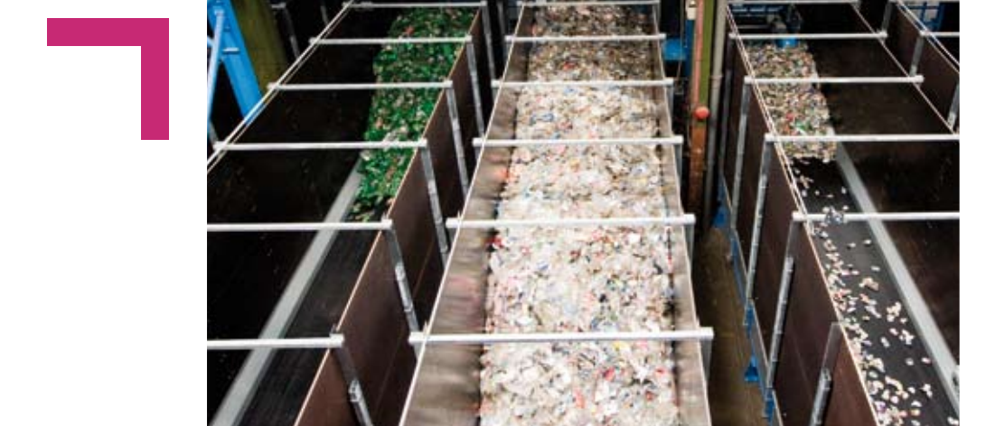
Bunker conveyors with separated fractions
